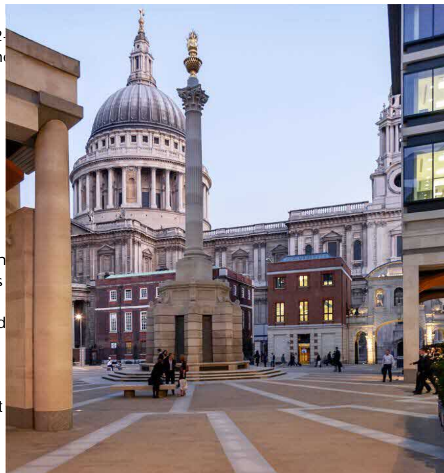
Paternoster Square looking to the drum, dome and N transept pediment of the Cathedral (picture credit: Historic England).
