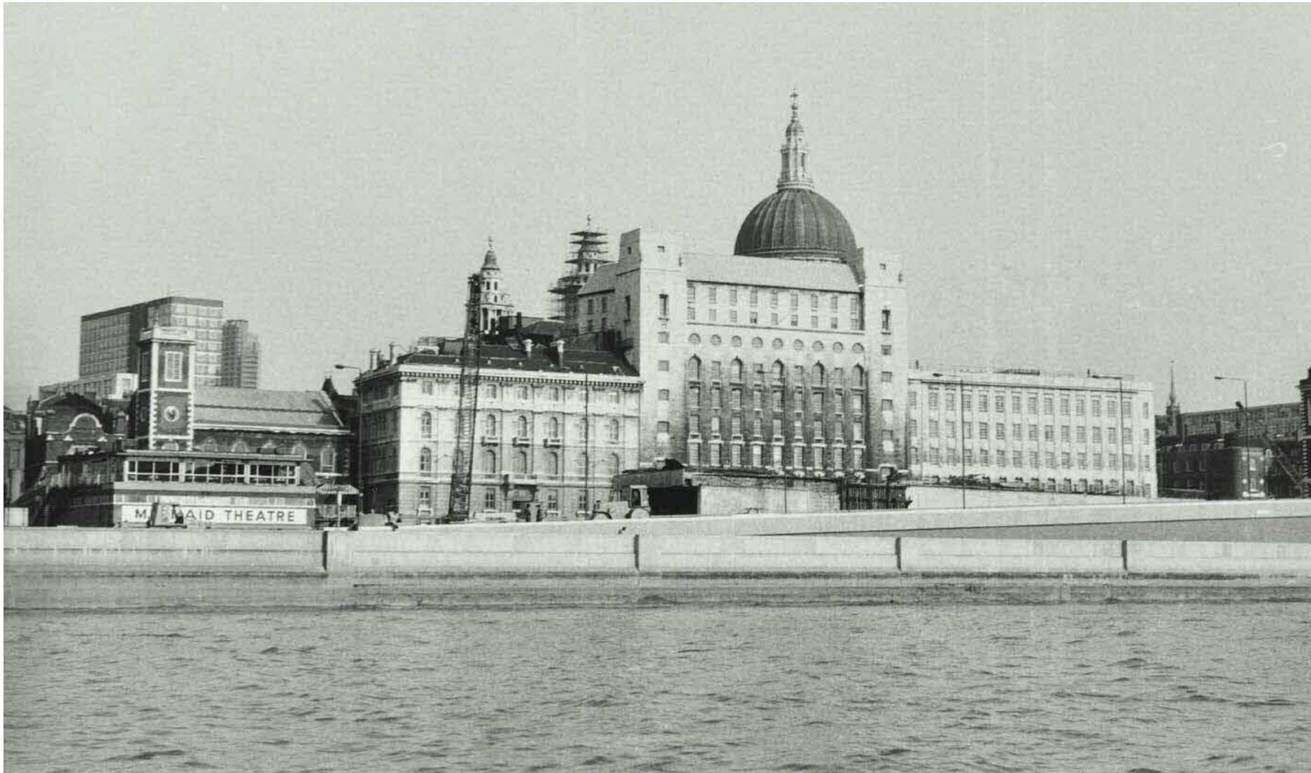
A photograph of the Faraday Building taken from the river in the 1950s, which illustrates the impact the building had on views and the setting of St Paul's (picture credit: © London Metropolitan Archives, City of London).
